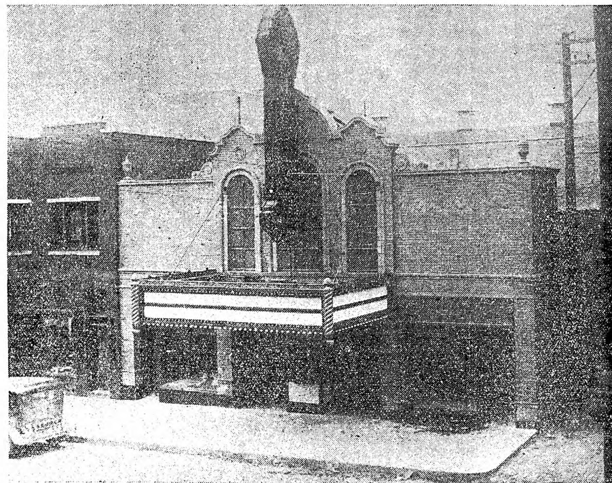
Exterior view of the Patio, Freeport's new amusement house, which will open to public patronage tomorrow. The front is of buff brick and terra cotta and architecturally of Spanish adaptation. While modest in appearance a mere glimpse of the lobby gives promise of the gorgeous and colorful interior of the theatre.
