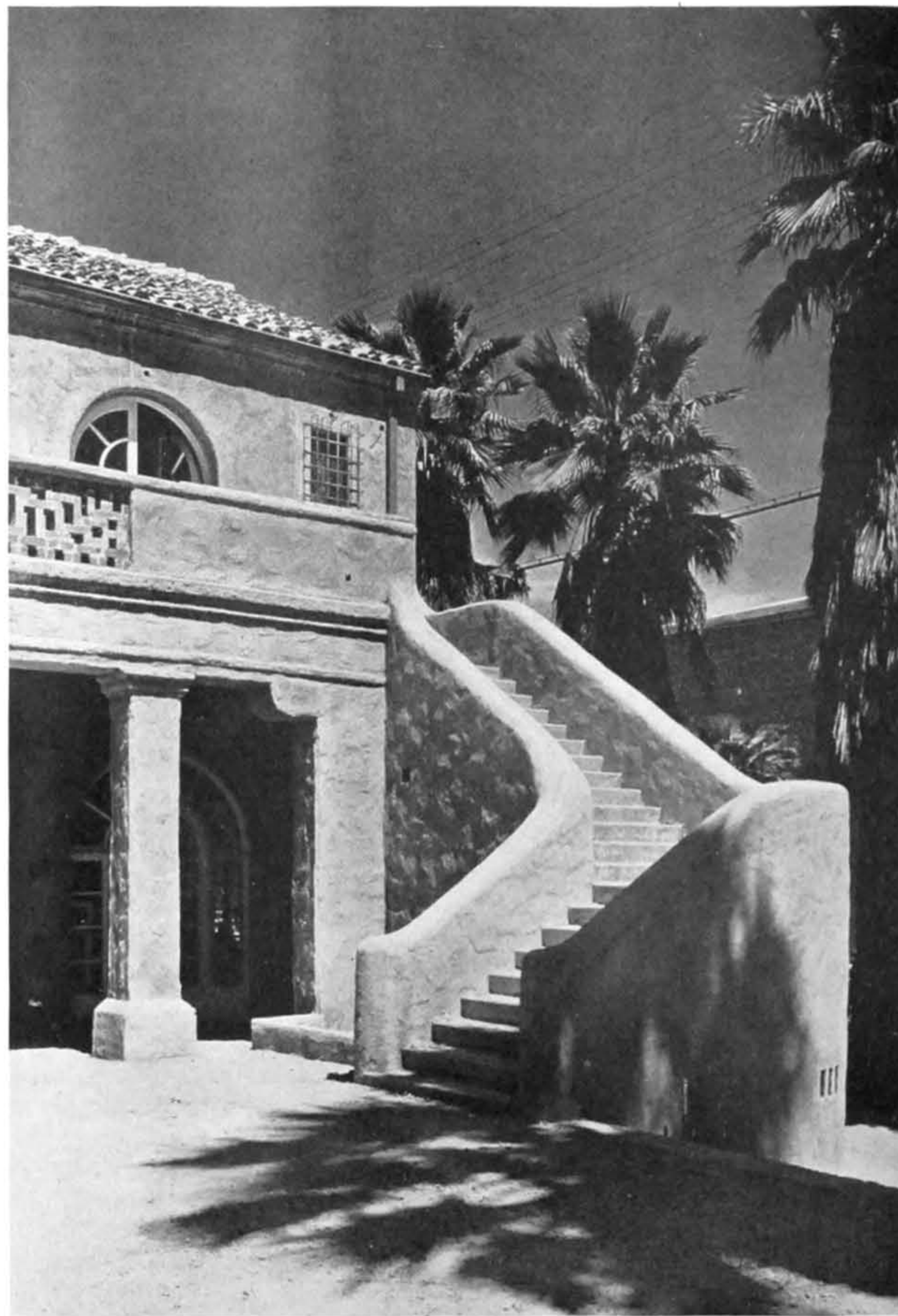
THE STAIRWAY TO THE MUSIC ROOM WHICH AWAITS COMPLETION.
