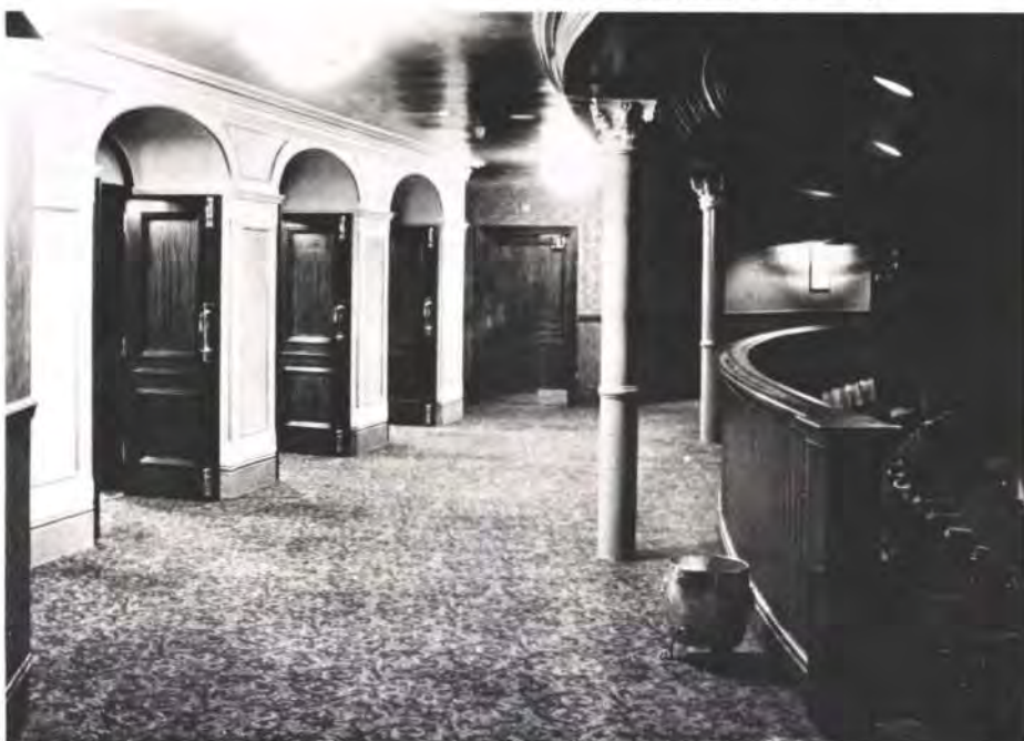
Fig. 12 The 1st tier, showing soffit lights and the fibrous plaster profiles which mark the air distribution outlets
